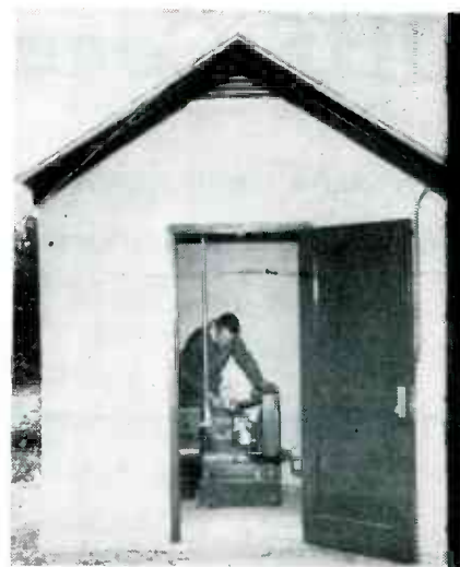
Emergency power stations at each relay position insure communications in the event of regular power system failure
