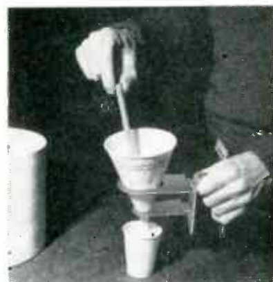
Demonstrating Emerson's use of conical paper cup and dowel-rod valve for filling containers with potting compound. Military classification prevents showing actual component. Compound is mixed in gallon icecream container at left
