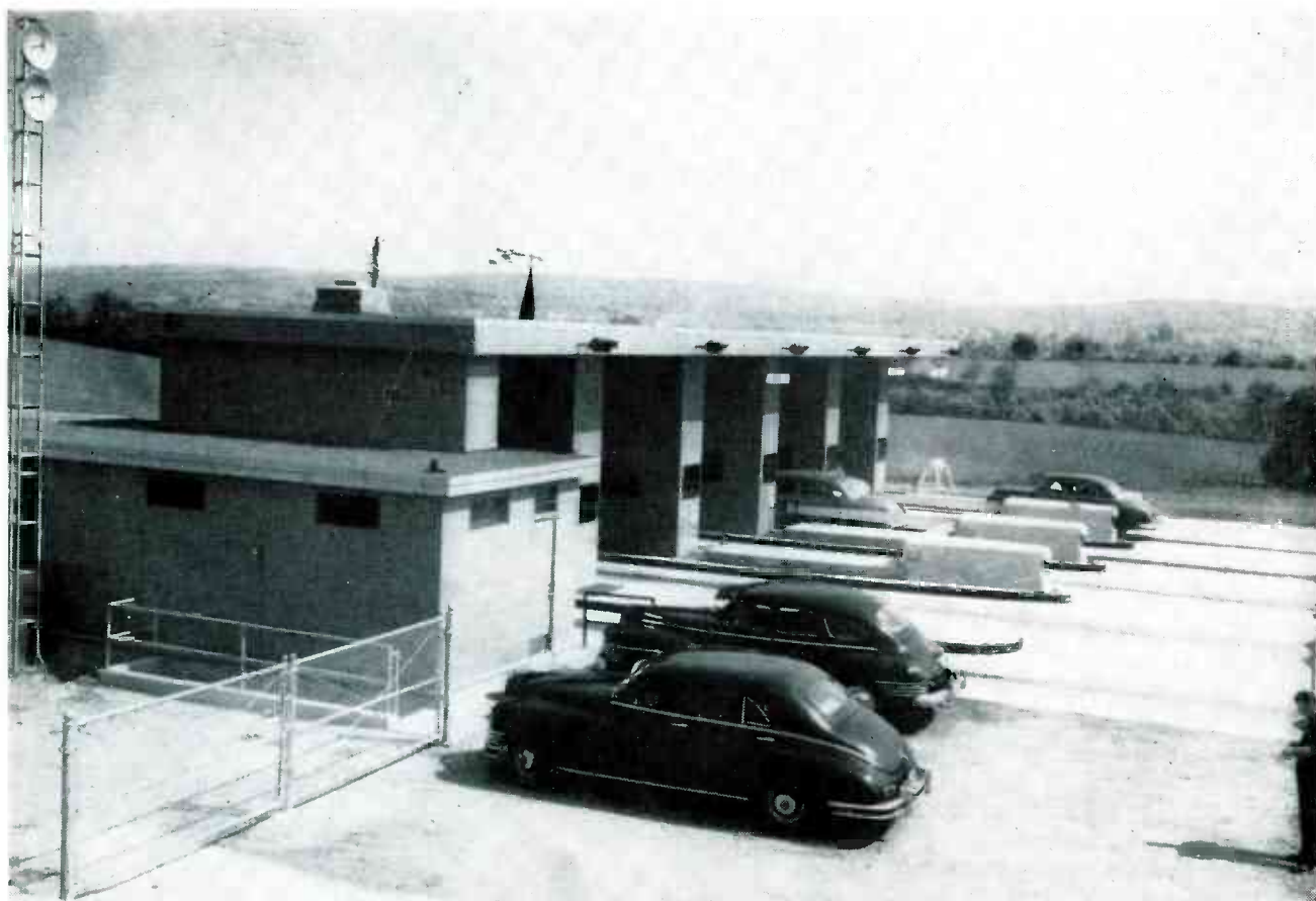
Valley Forge interchange, eastern terminus of the Pennsylvania Turnpike, is also eastern end of microwave system, as indicated by one-way set of parabolas in upper left-hand corner of photograph
