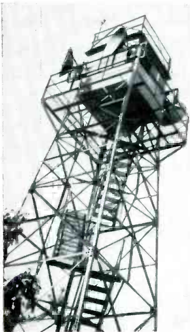
Thirteen two-way microwave relay stations of the type shown furnish dependable communications along the route. Average hop is 24 miles
